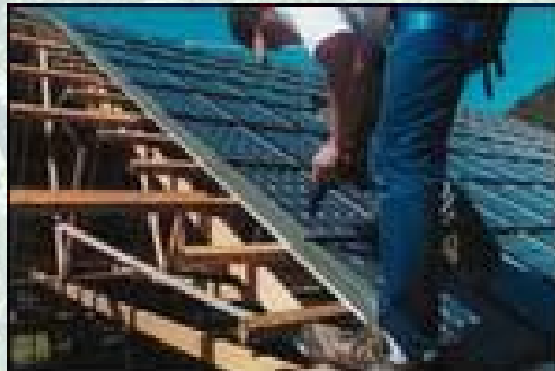
BiPV being installed
