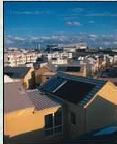
1kW BiPV (plus solar hotwater) at Newington
