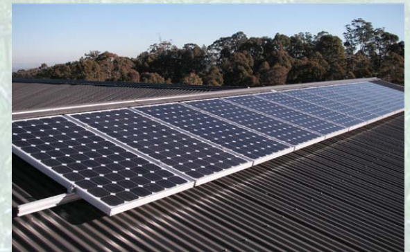
2kW crystalline cells
